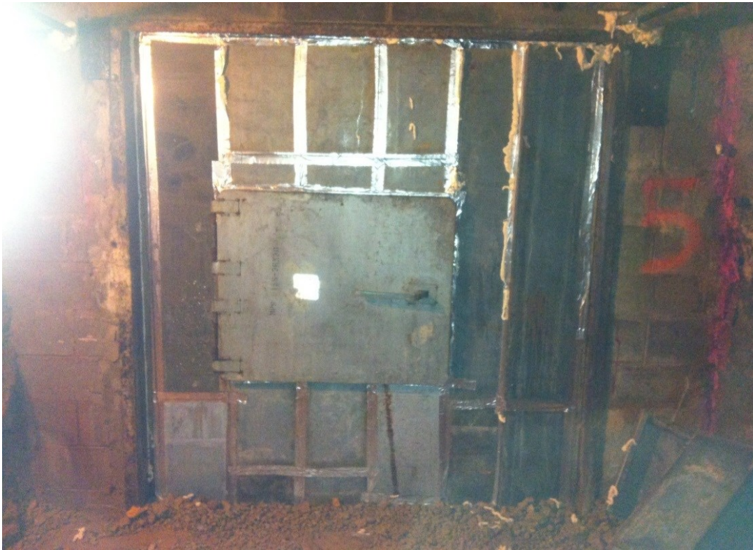
Figure 3.16 Kennedy steel door
